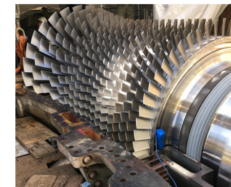
PSM seed rotor installed with new row 9-17 compressor wheels
